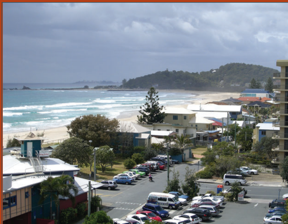
figure co.1 The joys of living beside the beach—sun, sand, saltwater and corrosion!
