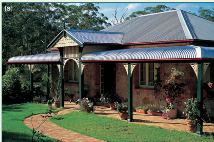
figure co.11 (a) Galvanised iron roofs are common throughout Australia. (b) The iron is protected as the zinc coating gives up its electrons.
