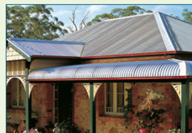
figure ec.5 Galvanising iron by electroplating protects the iron underneath from corrosion. Galvanised iron is commonly used as roofing.
