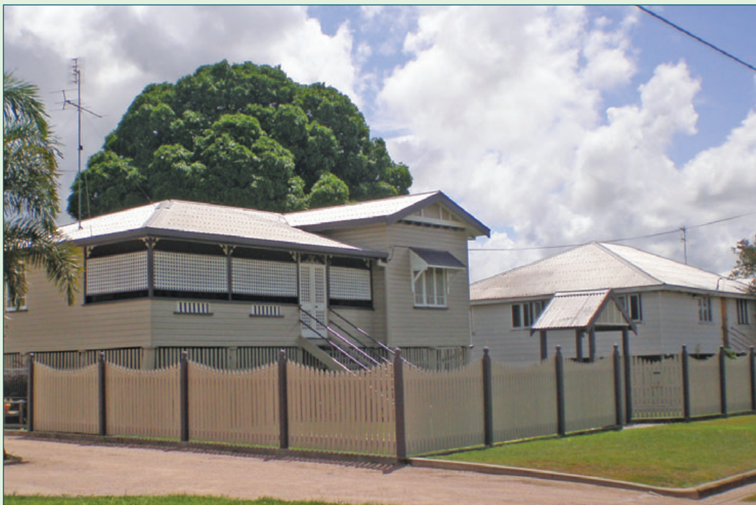
figure mn.6 Galvanising with zinc protects this roof from rusting.
