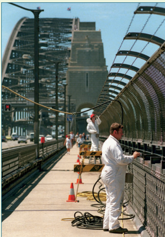
figure co.10 The Sydney Harbour Bridge is a 53 000-tonne steel structure protected from corrosion by paint. This is a continuous process that uses 90 000 litres of paint per coat.
